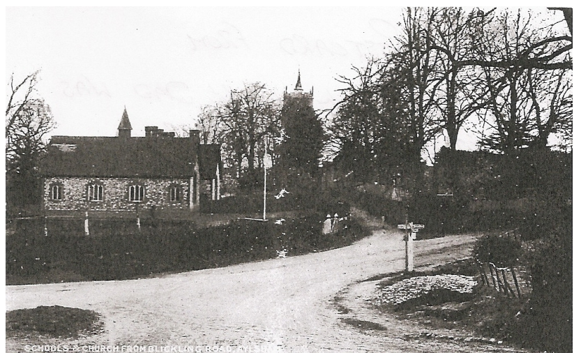
Schools and church from Blickling Road
