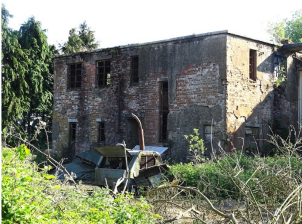
The old Control Tower complex at RAF Swannington in May 2018.
