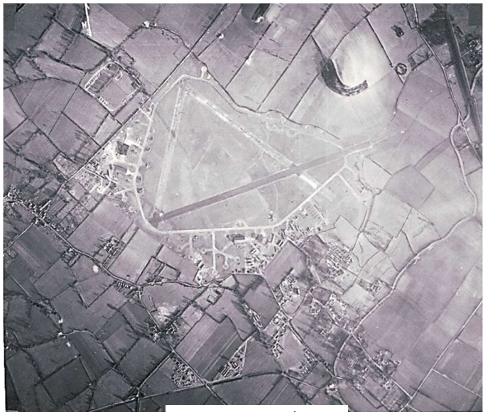
Stn. 113 Aerial View
