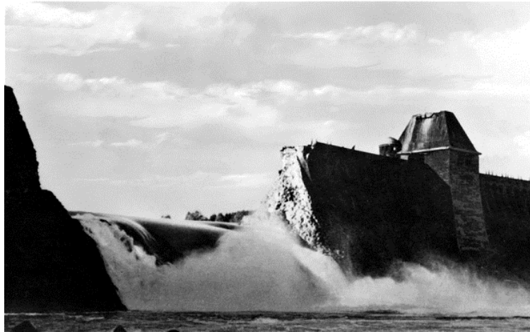
The damaged Mohne Dam in the Ruhr Valley after the RAF Dambusters raid Photo: Alamy
